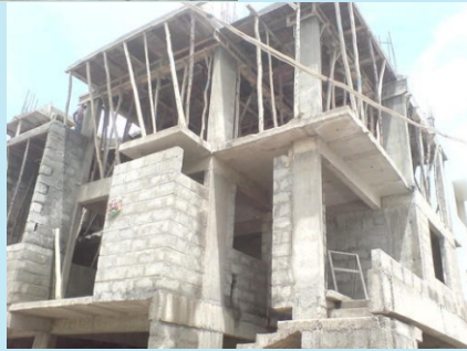
Mukti Sikha Ashram Building During Construction Stage in 2011 At Rajarhat
